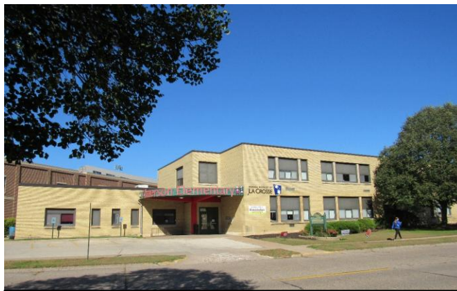
View of the modern main entry at the southwest corner of Emerson School. October 2025.
