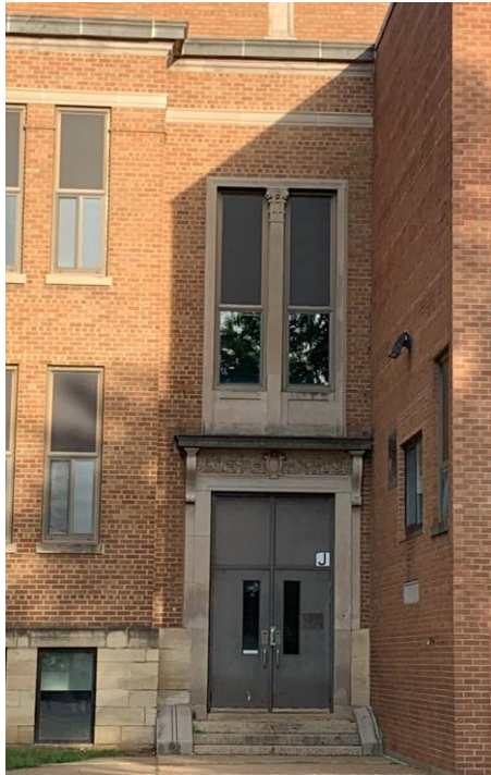
Marc Zettler photo: Detail of front doors, south pair, at the west façade of Hogan School. September 2025.
