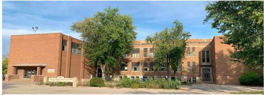
Marc Zettler photo: View of west (front) façade of Hogan School. September 2025.
