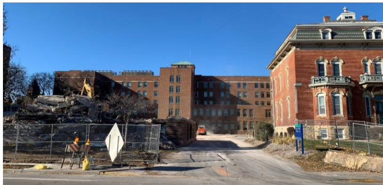
View of the west façade at the School of Nursing. During the St. Ann’s demolition. November 2025.
