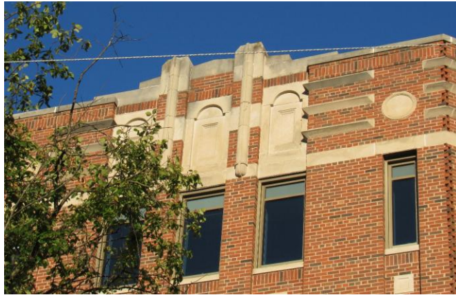
Detailed view of the parapet detail above the main entry at the School of Nursing. October 2025.
