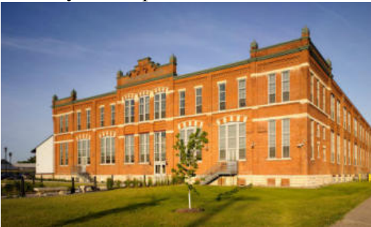
Gund Brewery Loft Apartments
